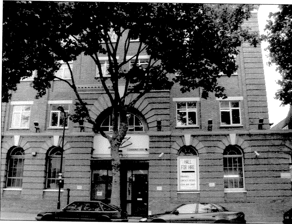
Figure 6: Live / Work at No.28 Lawrence Road
